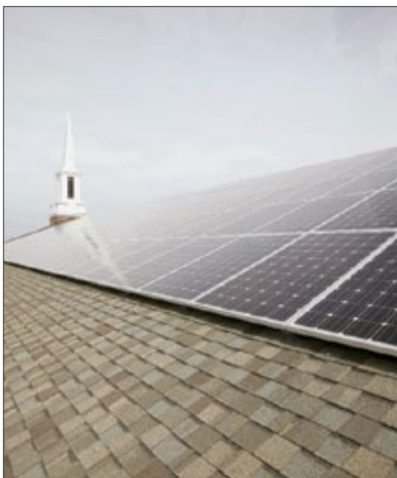
Solar panels were installed on the Farmington meetinghouse roof.
